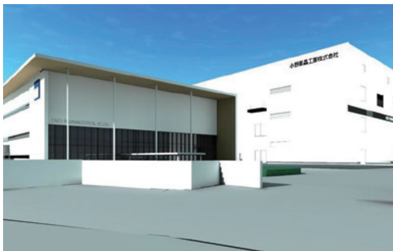
As-built image of Yamaguchi Plant
